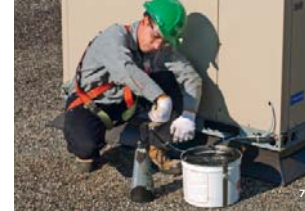
SEALANTS SHRINK AND CRACK OVER TIME. REAPPLICATION ENSURES INTEGRITY [7]. CLEARING ROOF DRAINS IS PART OF ONGOING ROOF MAINTENANCE. [8].
