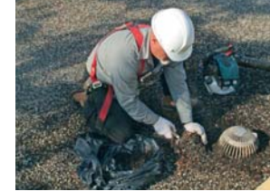
SEALANTS SHRINK AND CRACK OVER TIME. REAPPLICATION ENSURES INTEGRITY [7]. CLEARING ROOF DRAINS IS PART OF ONGOING ROOF MAINTENANCE. [8].
