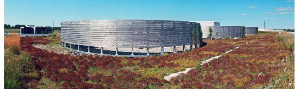
THE ACCELERATOR BUILDING IN WATERLOO WHERE A VARIETY OF PLANTS CREATE A MEADOW-LIKE EFFECT. THE ROUND WOOD STRUCTURES ARE SCREENS TO HIDE THE ROOF-TOP MECHANICAL EQUIPMENT [3].
